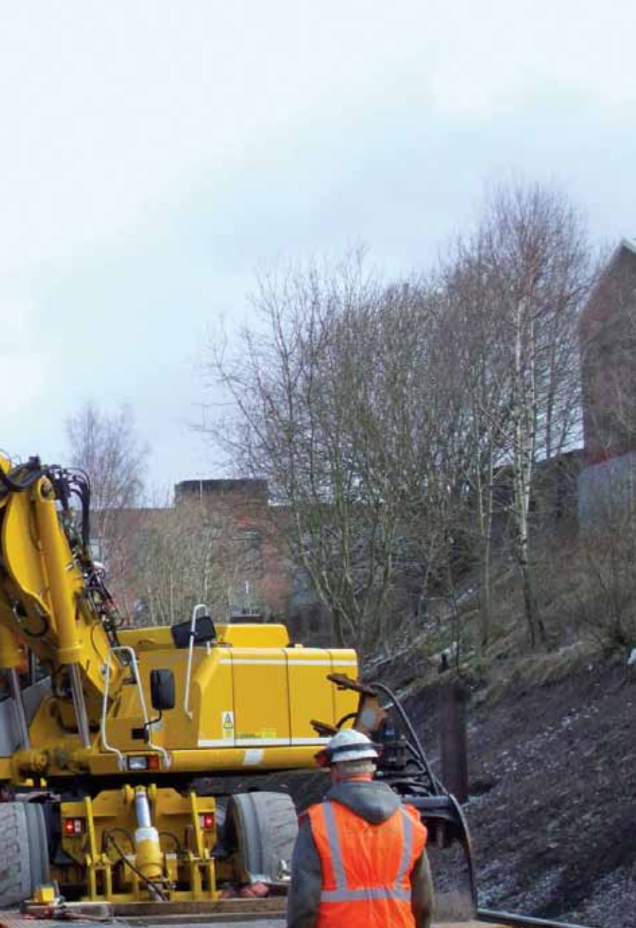
Main Image: BSP DX-RT 25 driving railway electrification stanchion piles, Manchester, UK
